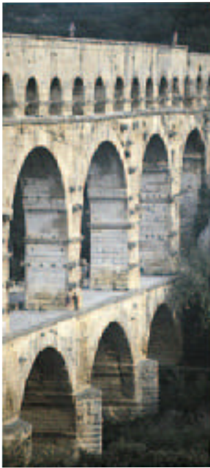
PONT DU GARD, FRANCE A vast stone three-storied bridge carried an aqueduct over a gorge. The water flowed through a covered channel along the top. The aqueduct ran for about 30 miles (50 km), ending in a reservoir which supplied 20,000 tons of water to the city of Nimes every day.
